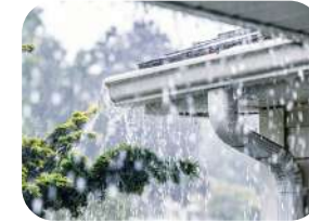
Rain Water Harvesting
